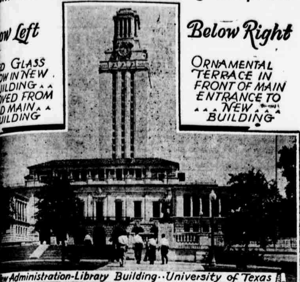
Administration-Library Building—University of Texas
