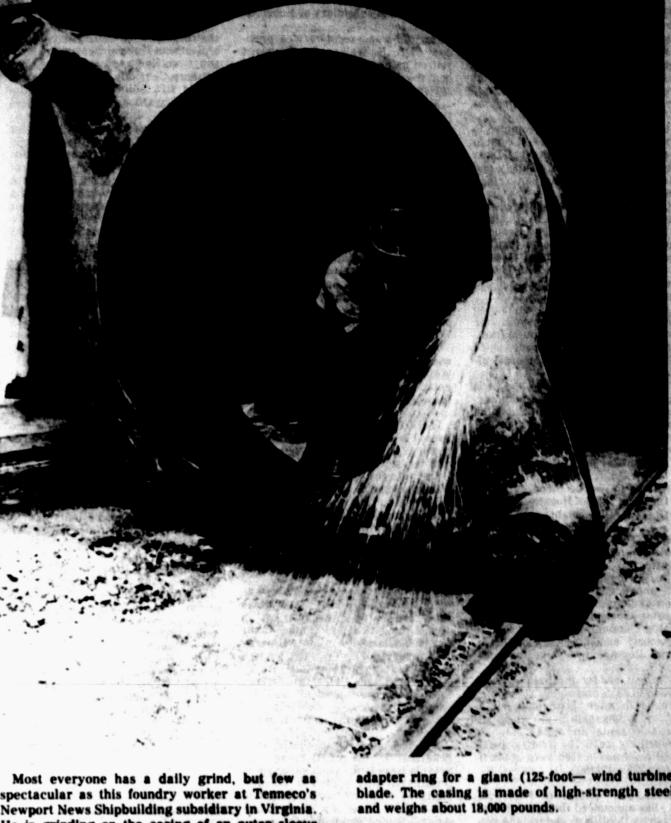
spectacular as this foundry worker at Tenneco's Newport News Shipbuilding subsidiary in Virginia. He is grinding on the casing of an outer sleeve adapter ring for a giant (125-foot- wind turbine blade. The casing is made of high-strength steel
