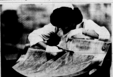
The plastic bagging material is cut away, exposing the newly shaped graphite "fabric," now hardened by heat and pressure.
