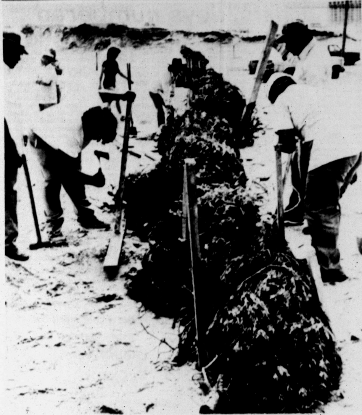
Cameron County workers build a 300-foot-long fence of Christmas trees at Andy Bowie County Park recently as part of a project to rebuild sand dunes that were flattened in August by Hurricane Allen. (AP Laserphoto)
