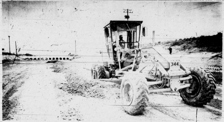
Scraping dirt as it goes westward, a piece of heavy equipment dredges the Northwest Drainage Channel to widen and deepen it in one of the city's major projects. When com-
