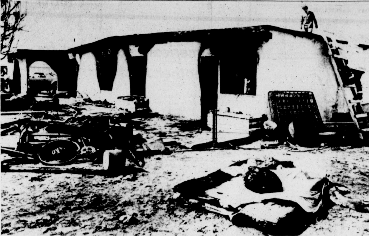
Fire Marshal Joe Wilson climbs onto the roof of the de la Rosa family home in El Paso, where three children died in a fire. Wilsom blamed the fire on faulty electrical wiring and said firefighters were hampered because the adobe
