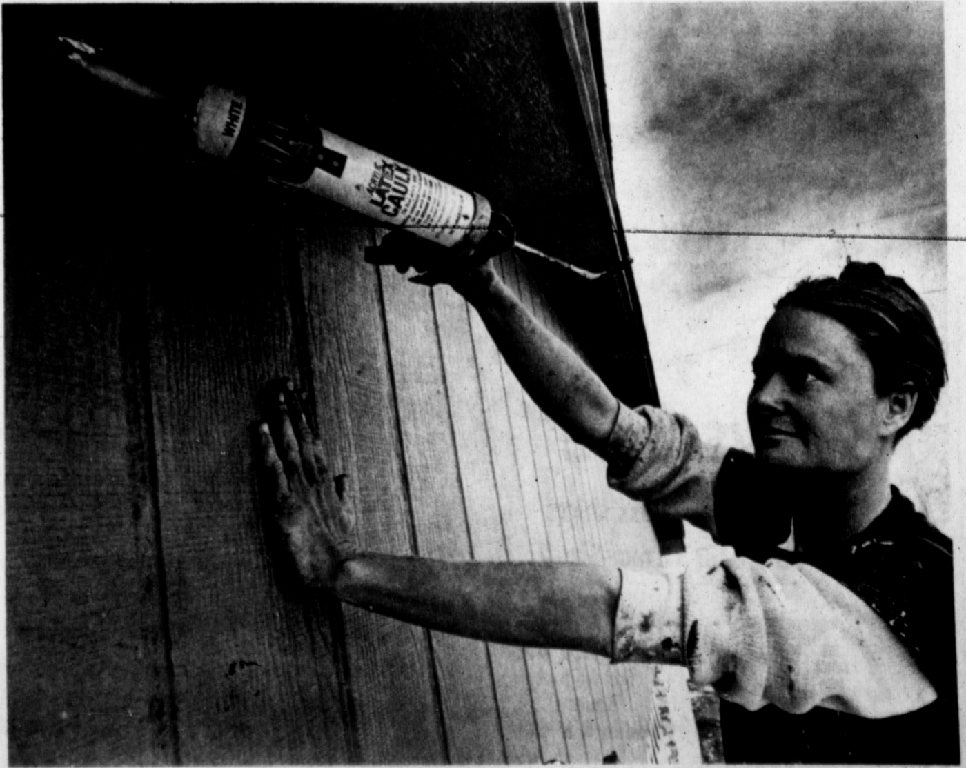
Vicki Behl applies caulking to a roof overhang to insure insulation.
