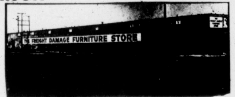
2900 WEST FRONT ST. THE BIG PURPLE BUILDING
