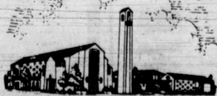
First United Methodist Church Main Street at Illinois Avenue Midland
