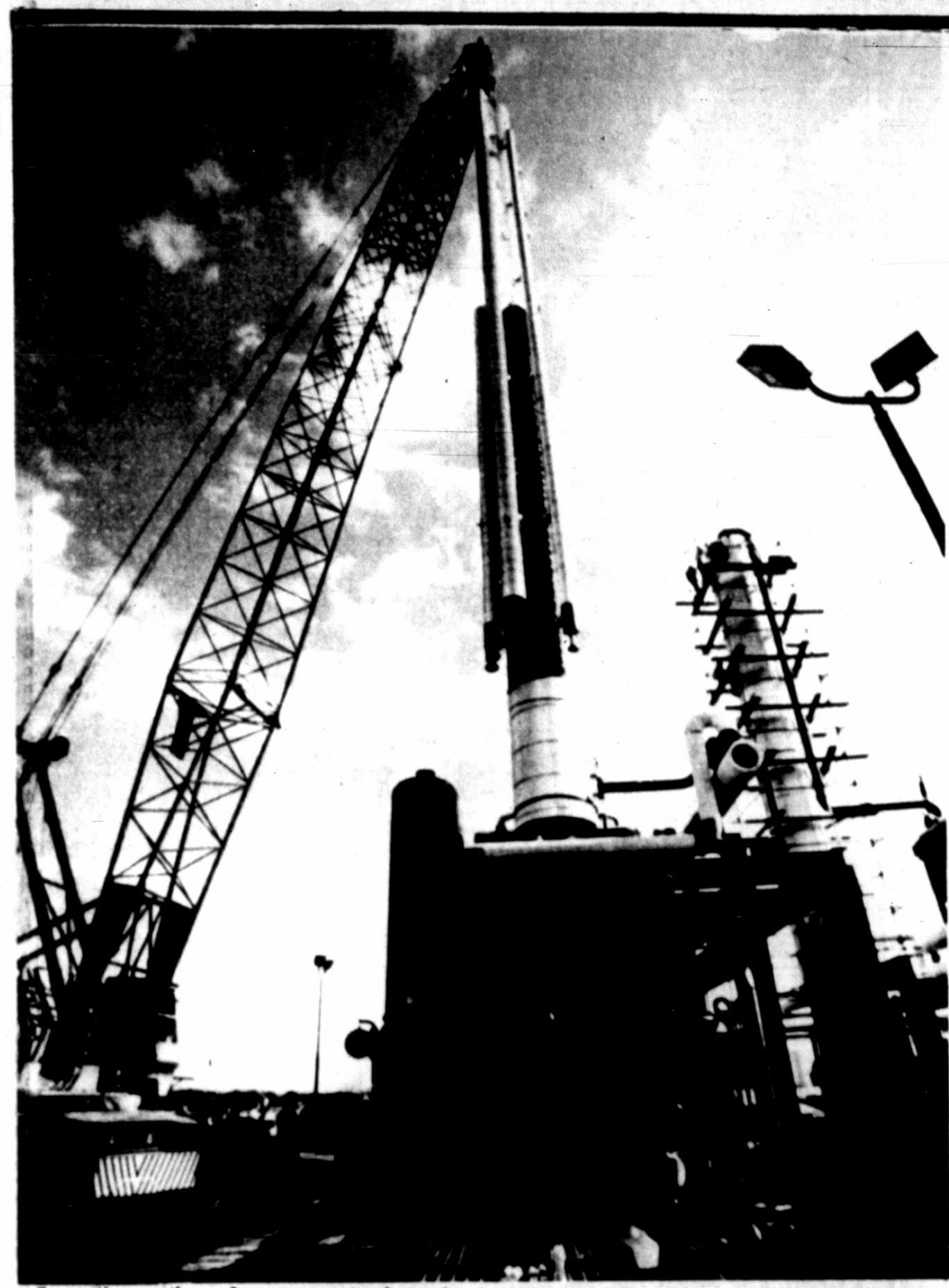
Separating methane from raw natural gas is what this 100-foot high "demethanizer" will do at this new 50-million-cubic-foot-per-day capacity processing plant in Live Oak County. Operated by Aminoil USA, Inc. in partnership with El Paso Natural Gas Co., the plant is designed to separate gas into liquid products from Aminoil's East Chapa field, in addition to gas from other producers in the area.
