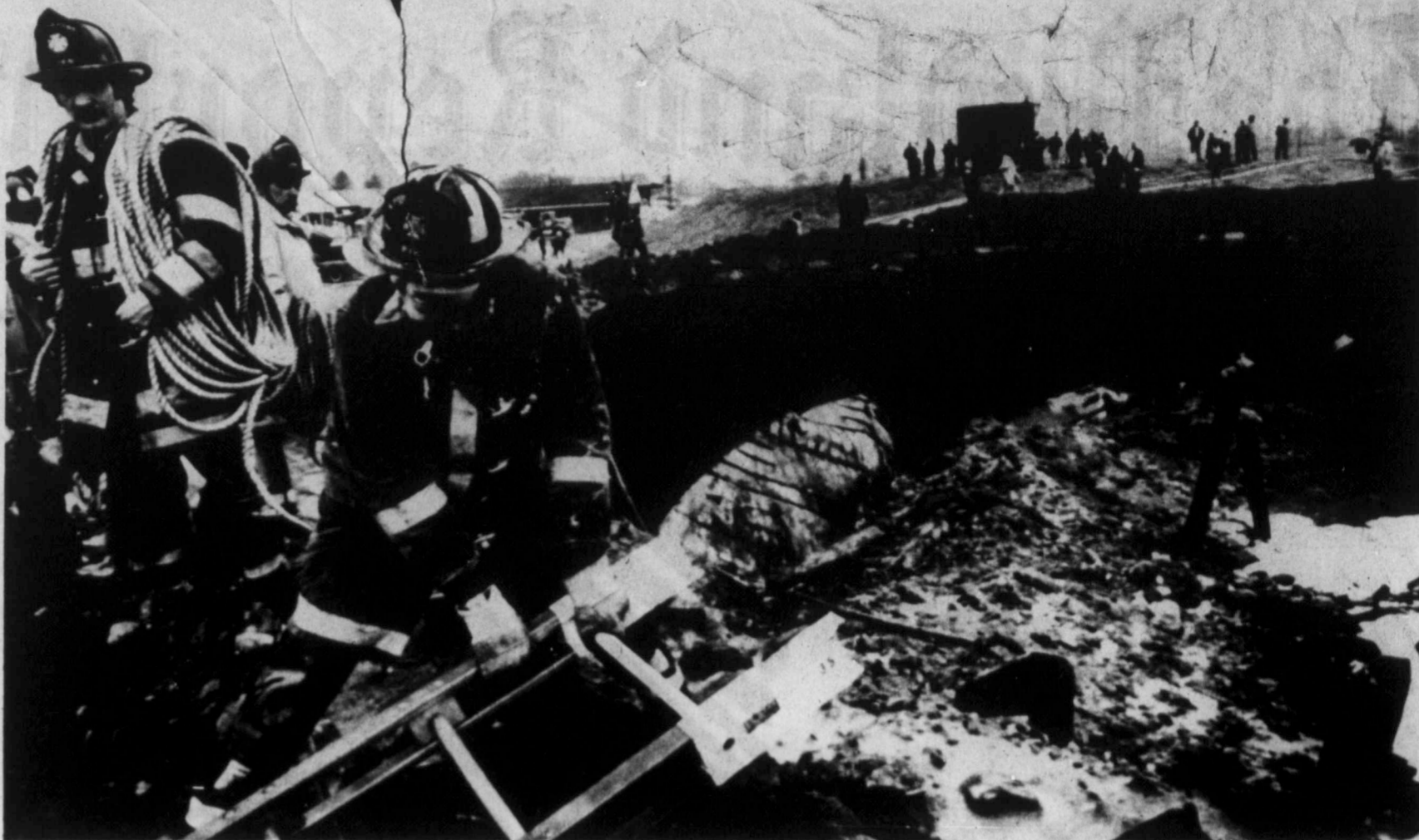
Firefighters prepared Wednesday to climb down into the crater left by the explosion and collapse of a huge jet fuel storage tank cleaned
