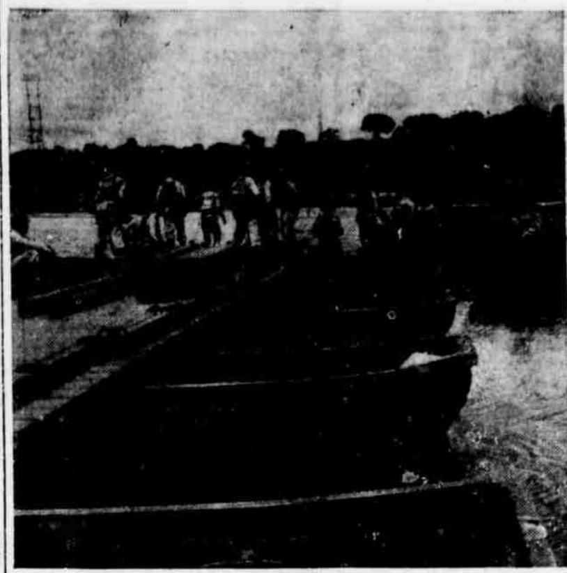
Army engineers in the Canal Zone set what is believed to be an all-time record by spanning a river with a 1,070-foot pontoon bridge in one hour and 40 minutes, in a test to show how they could span rivers under fire. The last section here is swung into position ready for a test run of a ten-ton unit.
