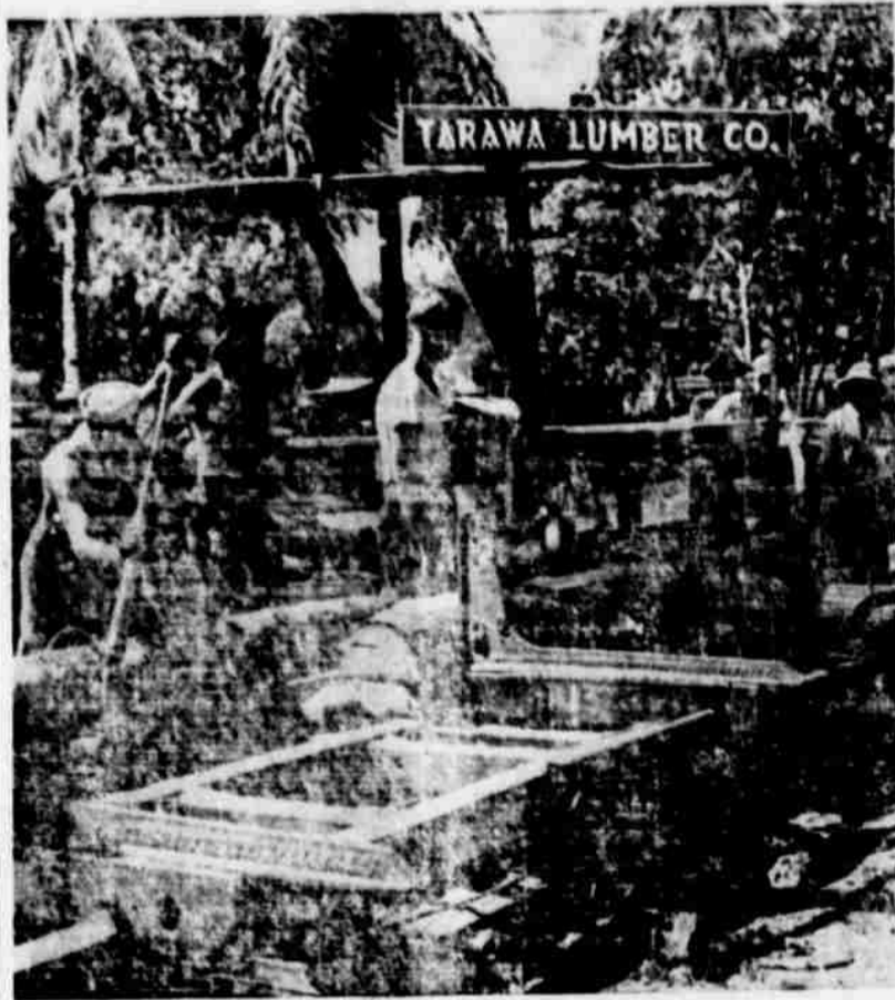
This sawmill was imported to Tarawa to aid in the reconstruction of the former Japanese base after the marines took it in the bloodiest battle of their history. The mill turns out lumber for tent frames, flooring and many other uses. The navy seabees and marine engineers have done a masterful job in improving this important Gilbert Island base.
