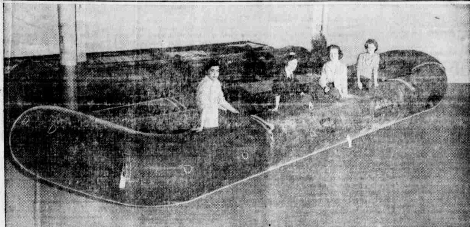
In all quarters of the globe U. S. Army engineers are throwing ponton bridges across streams to carry the troops and equipment of the fighting forces. This new ponton has been developed with turned up edges to give more stability to the ponton and to prevent capsizing...
