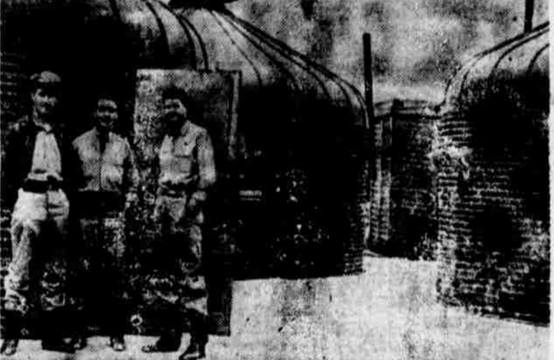
These metal buildings in Iran were formerly used for storing grain. Now they serve as officers' quarters for U. S. forces in that country. Three tenants standing outside their peculiar homes are, left to right Captains B. E. Seitzinger, Fairfield, Iowa; J. W. Cofer, Louisville, Ky; and R. L. Clayton, Minneapolis, Minn.
