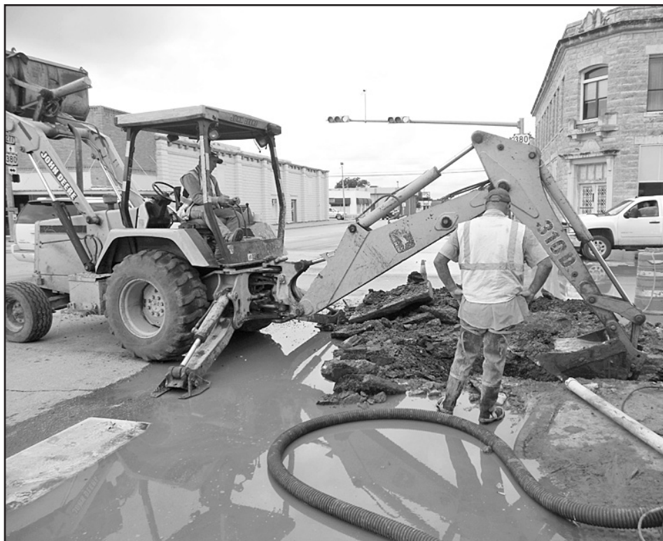
WATER LEAK —Crews were working to repair a water leak in an eight inch pipe at the intersection of Hwy. 380 and Hwy. 277 in downtown Haskell Monday. The repairs began Friday with the replacement of a fire plug that was damaged in a truck accident in June. Further woes occurred when it was discovered that the main pipe was also leaking.
