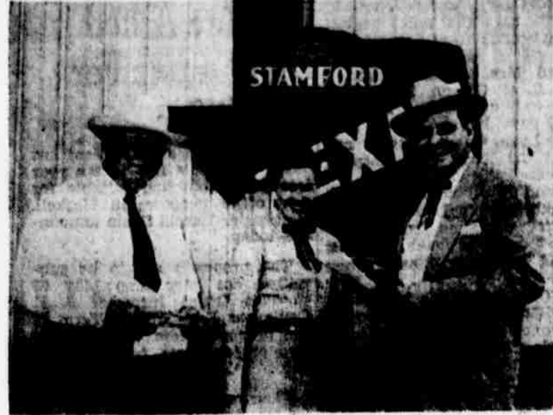
Stamford celebrated the formal opening of its first manufacturing concern, a western clothing firm, with an all day "Open House" Saturday. Standing before the air-conditioned building that houses the Feldt Manufacturing Co. are Stamford's Mayor G. C. Carothers, Official Hostess Miss Jan Crafton, Max Feldt, pres.
