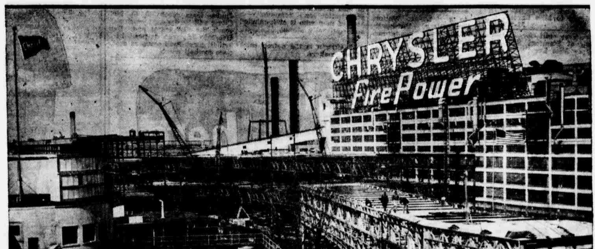
UP GOES CHRYSLER'S PRODUCTION MORE THAN 40% Here you see construction work proceeding on the new Chrysler production facilities which will add 667,000 square feet of floor space . . . including a 14-mile long continuous conveyor system, longest in the industry.
