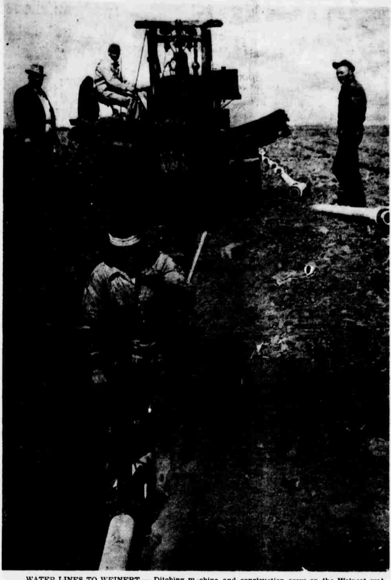
WATER LINES TO WEINERT — Ditching machine and construction crew on the Weinert waterworks project pictured here has almost completed laying the main supply line from wells to the city limits. The pipe is being laid in a ditch 3 1/2 to 4 feet deep, and the machine digs from 600 to 800 feet of ditch per hour. In the picture at left is S. E. Lanier, contractor; John C. Hill, ditching machine operator; in foreground in W. J. Turnbow, m.k.ing pipe connection; and standing at right is Charley Hix, member of the construction crew. (Photo by Blohm)
