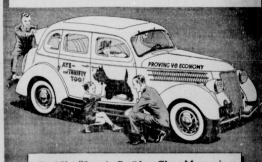
Ford V-8 "Scottie Car" has Glass Measuring Tank - shows Exact Gas Consumption
