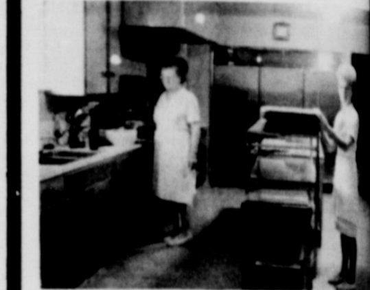
Pictured above is the Total Electric Kitchen of the Care Home.
