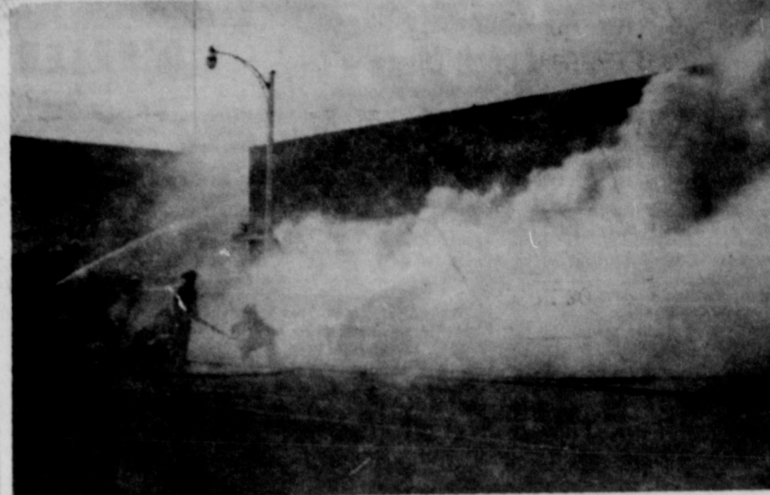
Smoke boils from the front of Lewis Building and just about covers fire fighting equipment and firemen during a two hour battle that wiped out the largest downtown building in Knox City. (Staff Photo)
