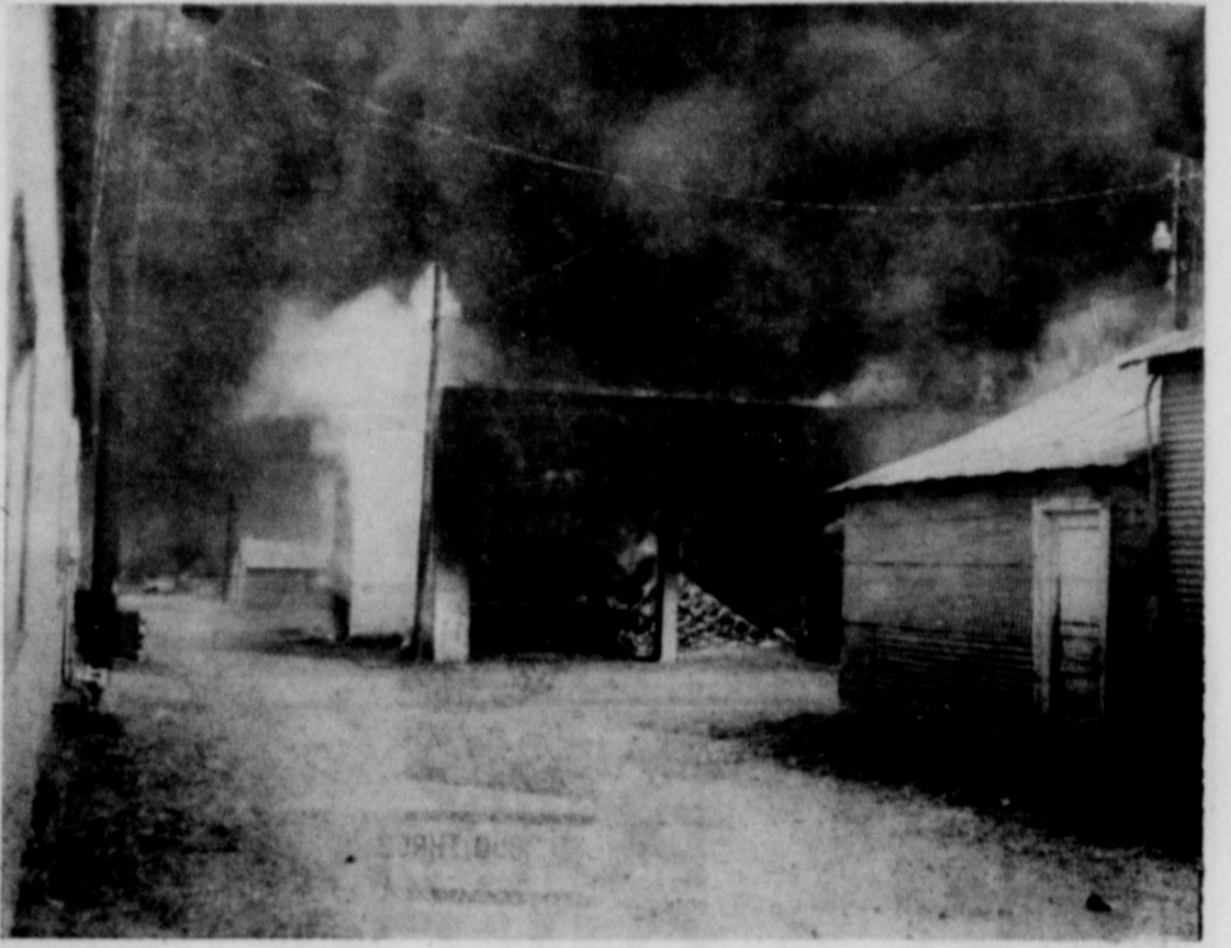
Three cars are airtie in the back shop. Eddie Singleton and Jimmy Parker drove two pickups, two passenger cars and the company wrecker out before the flames took the building over. (S-Photo)
