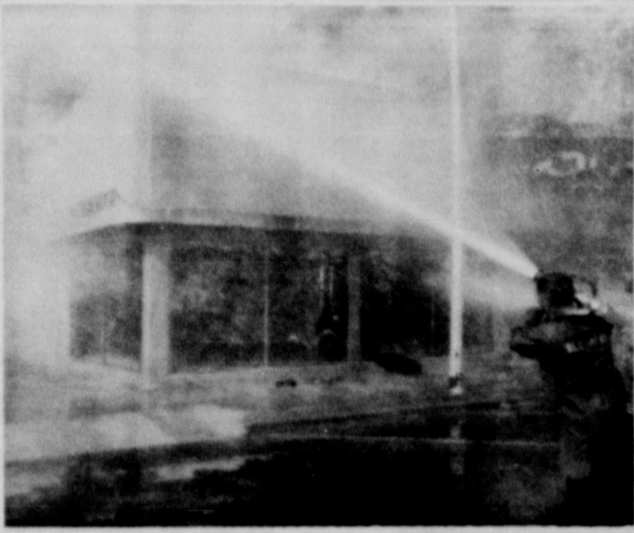
Front of Lewis Building was still standing and some plate glass window are in place — but the inside is "gutted" and roof beams are falling in. (Staff Photo)
