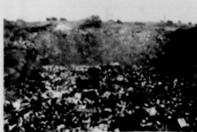
KNOX CITY SANITARY Landfill. In the background garbage has been rolled and packed with soil material. The dumped garbage in front will be covered with 6 to 8 inches of soil and pushed back to the pit area and covered.
