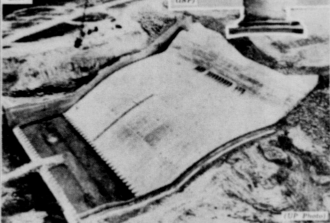
SPILLWAY of new $19,500,000 Kirwin Dam near Phillipsburg, Kas. looks like flowing front of old-style cash register.
