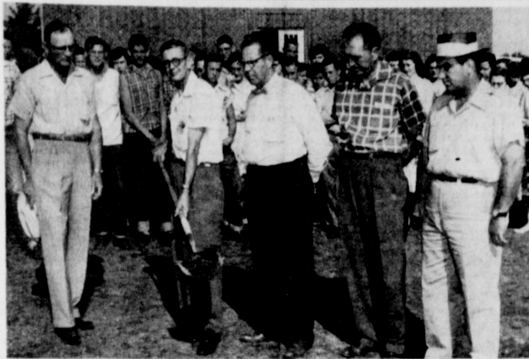
GROUND-BREAKING CEREMONY —Guy Robinson, president of the Knox City School Board, dug the first shovel-full of dirt Tuesday in preparations for construction of Knox City's new high school building. Looking on at left is Bobby Burnett, also a trustee, and at right are board member Horace Finley, Supt. Chas. E. Silk and J. C. Babb of Abilene, general contractor for the $153,360 construction job. Electrical work will be done by Graham Electric of Knox City, and Rowland Plumbing Co. of Vernon will do the plumbing and heating. Babb says the building should be ready for occupancy in 130 days.
