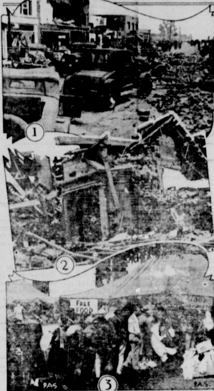
Here are photos from the heart of the earthquake zone which took 110 lives and did damage to property estimated at $50,000,000 in the Los Angeles area of Southern California. Photo No. 1 shows a street scene in Compton where 20 persons were killed by the collapse of building; No. 2, shows the ruins of a high school building in Long Beach, the town considered the quake's epicenter and where 45 lives were lost; No. 3, shows helplessness and penniless refugees being fed by the U. S. Marines at Long Beach.
