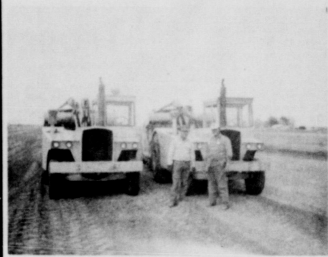
PICTURED above are two employees of Williams Tractor Co. and their machines, working on Knox City's Municipal Airport.
