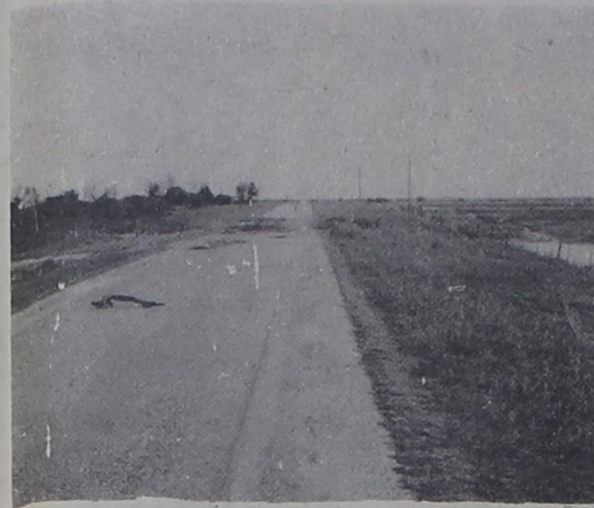
DEBRIS ON HIGHWAY: This debris deposited on Highway 222 near the J. D. Hicks farm home southeast of Munday, where Ricky Harlan lives, reveals that water ran across the highway at a spot where it was never seen before since the road was paved.
