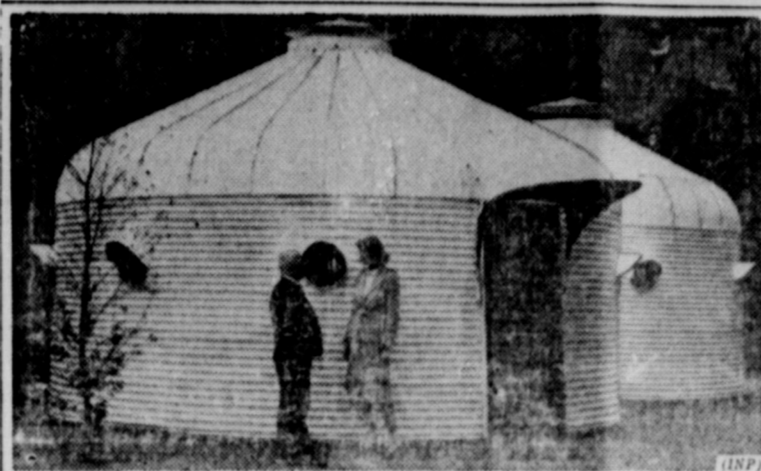
AIR RAID SHELTER —These circular structures of corrugated steel are new air raid shelters exhibited at Museum of Modern Art in New York. Inventor R. Buckminster Fuller (standing in front of shelter), says the shelters are also ideal for defense housing, troop barracks and beach houses. One of the advantages is the ease with which the units can be moved from place to place.
