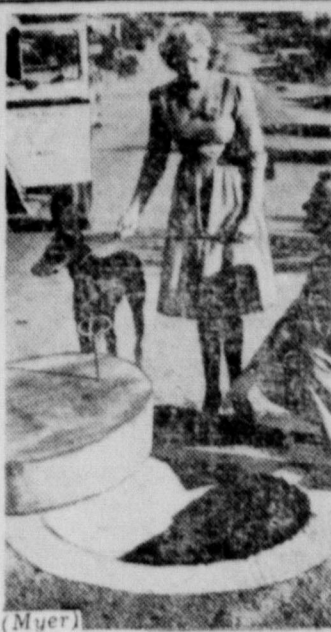
WOOD SUBSTITUTE —Los Angeles engineers built wooden manhole covers out of timbers treated to resist termites and decay when shortages threatened to delay sewage construction.
