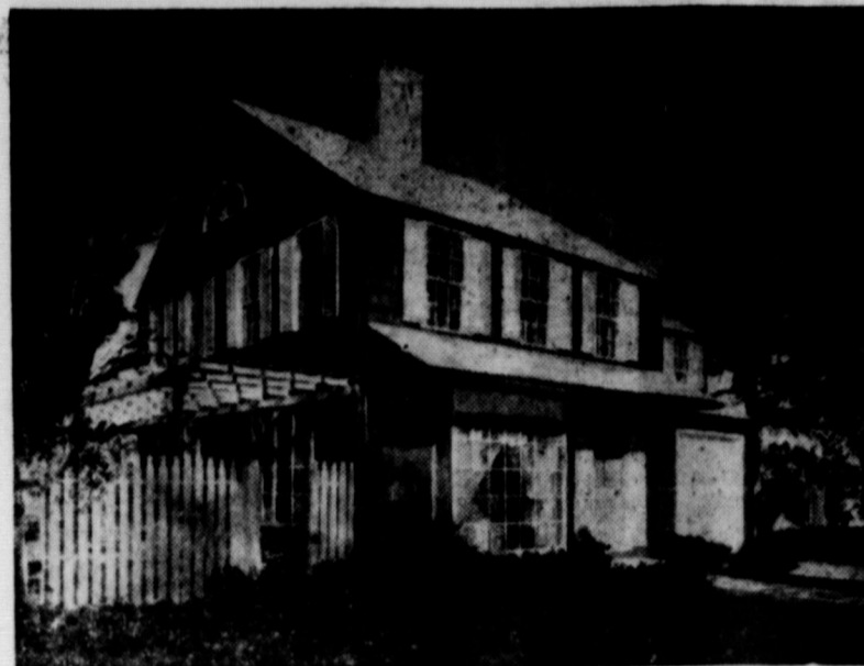
Add-on house forestalls those three unhappy results of attempting to build too much with too little money: undersized rooms, limited conveniences, compromised quality. Designed especially for the September issue of Good Housekeeping magazine, the add-on house starts life as a small two-bedroom home of only 17,500 cubic feet. When the budget permits, the 12½ foot wing with garage, laundry and bedroom may be added. Shown above is the street side with the solid assurance of its American lineage, dominated by a striking picture window.
