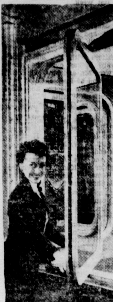
WASHING WINDOWS of the ultra-modern Alcoa Building in Pittsburgh, Pa., has been simplified by science. Washing the windows at Alcoa means deflating the butyl tube, swinging the window inside the building for cleaning, then swinging it back into position. The tube, designed by the General Tire & Rubber Company, holds the window in place. No longer need the window-washer dangle precariously from the 42-floor window casing. His is now an inside job.
