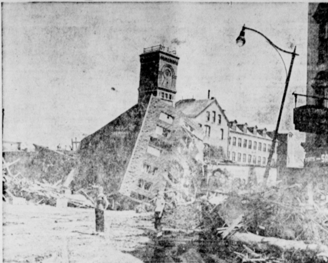
CRUSHED AND BROKEN , this 16-family apartment house in Waterbury, Conn., was left high and dry after the rampaging Naugatuck River receded August 21. This was a sample of devastation in the flood which, according to the Red Cross, destroyed 1,326 houses and badly damaged 4,805. (Wide World Photo)
