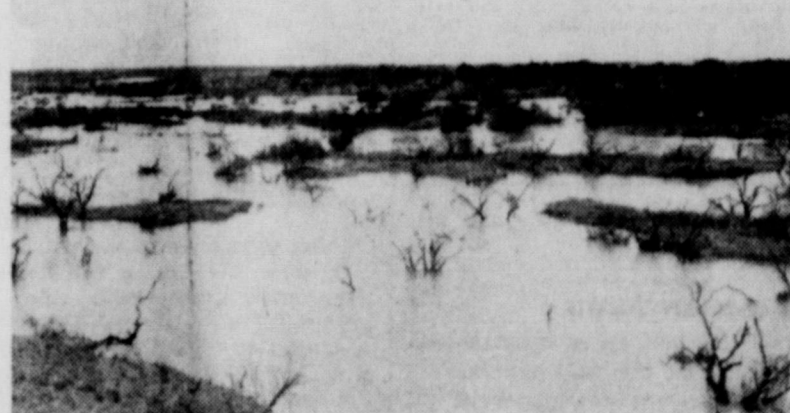
BACK WATER — From overflowing Miller Creek is shown here. Pond of water in upper left is some three-fourths mile from spot where picture was taken. Tall trees in background are along main channel of creek. Picture was taken Friday afternoon on C. P. Baker place, near the line of Haskell and Throckmorton County.
