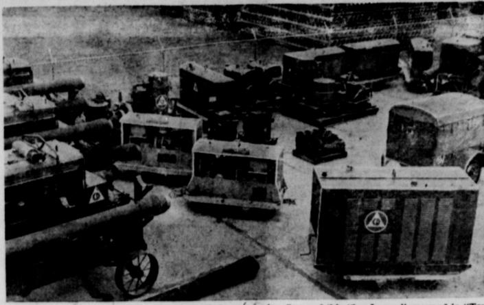
TYPICAL UNIT of civil defense stockpiling engineering equipment showing the pumps, generators, water purifiers, and some of the miles of flexible-coupled pipe which could be used after an attack to provide a stricken community with pure water. Some of this "hardware," grouped in "Ten-Mile Units" to service ten miles of pipe each, already has been used in natural disasters to pump out flooded areas, and to bring in and purify water for towns with dry reservoirs. (ODCM Photo)
