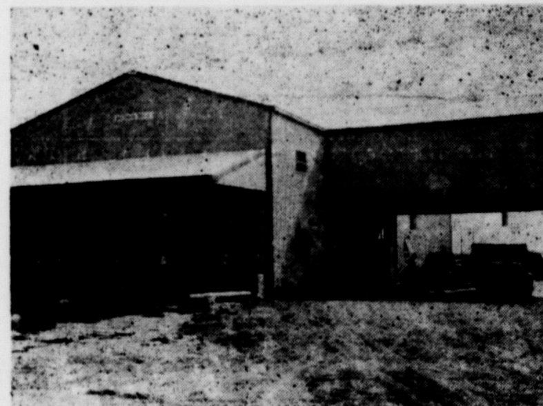
Exterior View of Our New Gin Plant
