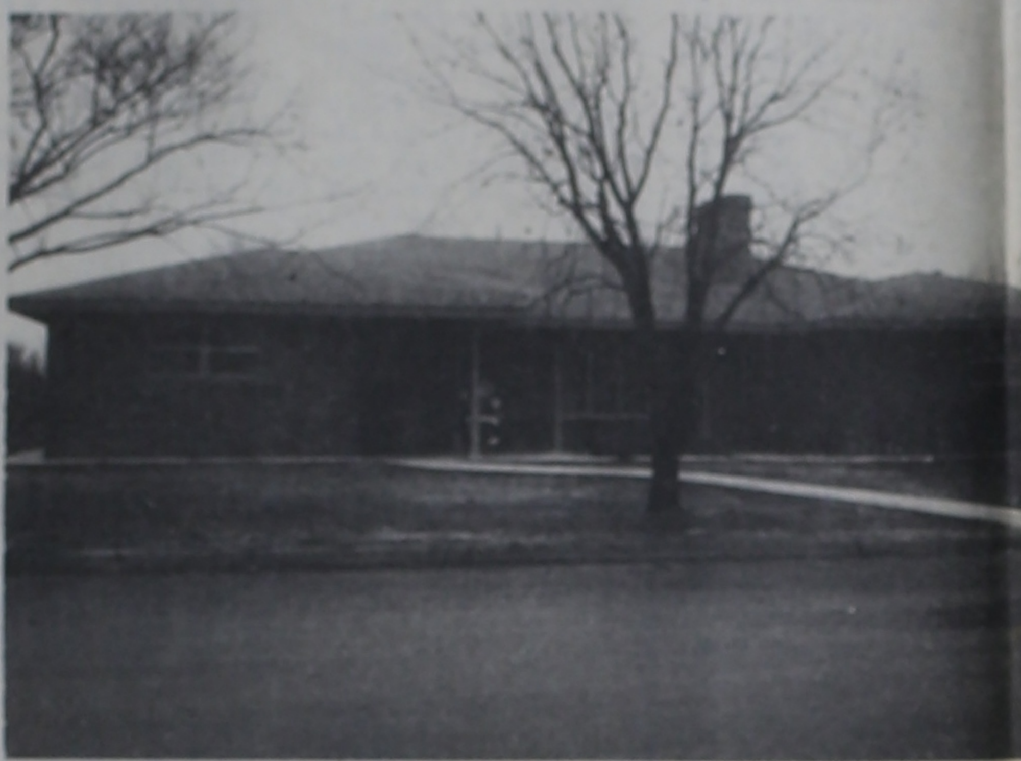
THE NEW HOME of Mr. and Mrs. Richie Smith, located on South 7th Ave., is one of the five new homes constructed in Munday during last year.
