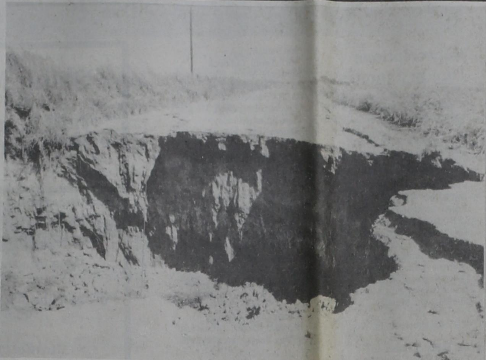
THIS COUNTY ROAD , heavily damaged by September rains, will be rebuilt and protected by a grade stabilization structure called a rock gabion designed by the Soil Conservation Service. Work on the road is expected to begin in February.
