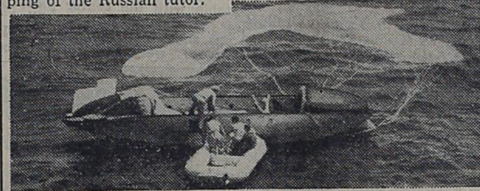
BOAT 'HITS SILK' in demonstration by Air Forces of dropping a two-ton metal rescue craft from a B-29. A parachute 100 feet in diameter lowered the boat, which has inboard motor, navigation devices and provisions for 15 men.
