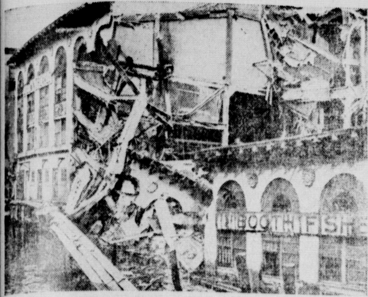
View showing the twisted mass of timbers after a 125-foot section of the Fulton Fish Market, for many years a landmark of the lower Manhattan waterfront, collapsed into the waters of the East river. This is the place where former Gov. Al E. Smith worked as a young man.
