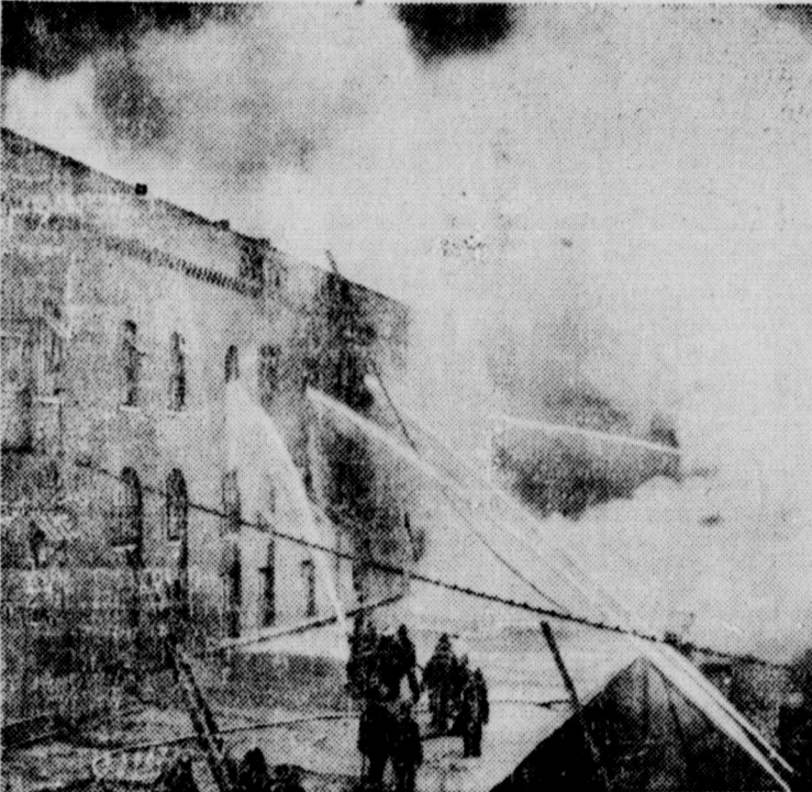
Flames which swept over a block-square building of one of the major meat-packing plants in the Union Stock yards at Chicago caused damage in excess of $200,000. Nearly a third of the fire-fighting apparatus of the city was called to the yards to prevent a spread of the conflagration. Picture shows firemen fighting the blaze.
