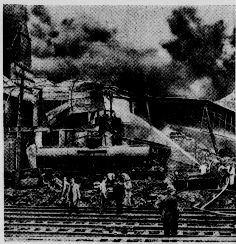
The burning ruins of two buildings are shown in the above photo of the Pennsylvania Industrial Chemical corporation at Clairton, Pa., which was damaged by an explosion of resin and oils. The blast resulted from "adverse chemical reaction" in an agitator. Six persons were injured in the blast. The damage is estimated at $50,000. Flames were brought under control an hour after the explosion.
