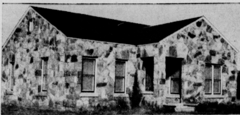
Pictured above is the home of Mrs. O. W. Orr and family, five and one-half blocks north of the court house square, which is owned and was remodeled last year by C. B. Graham. This was formerly the A. Brain residence. This native stone house contains five rooms and a bath.
