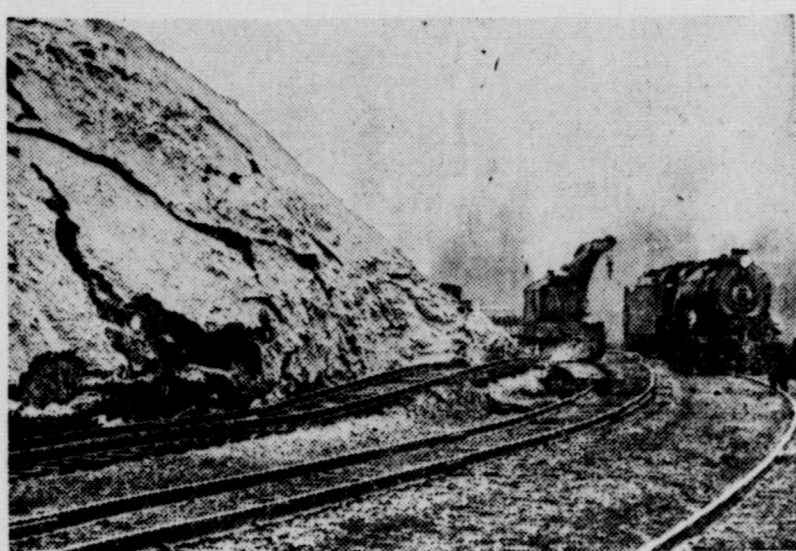
A landslide on the Conemaugh division of the Pennsylvania railroad along Pittsburgh's Allegheny River boulevard. An estimated million tons of dirt and rock slid down to disrupt rail traffic, and temporarily blocked the boulevard, one of Pittsburgh's main traffic arteries. Wheels of the freight engine were derailed.
