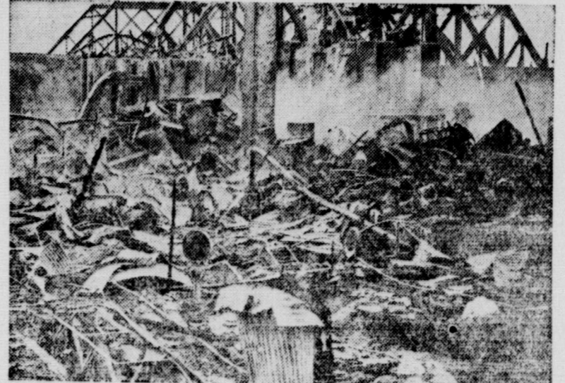
The FBI has started an investigation of the fire which totally destroyed the Exolon company abrasives plant at Bladell, N. Y., which was engaged in manufacturing defense materials. The fire caused damage estimated at more than a million dollars. Fire apparatus from Buffalo and surrounding suburbs helped fight the flames. Above is view of the ruins.
