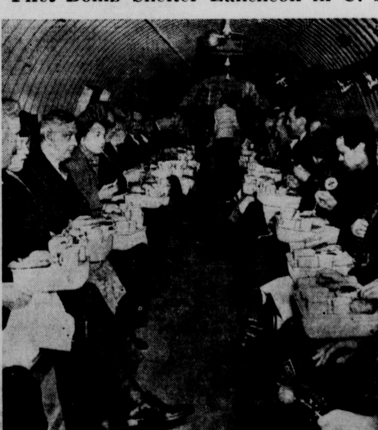
A luncheon served on air line trays publicly opened the bomb shelter by a large rubber concern at Akron, Ohio. This is a shatterproof flexible structure of the type tested by the war department. It is made of strong corrugated plates forming a gas and water-tight cylinder, and is large enough to accommodate 50 people.
