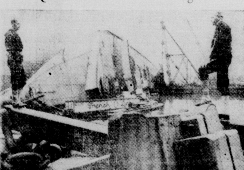
According to the report which Secretary of the Navy Frank Knox has given the President, the capsized former French liner Normandie, now the U. S. S. Lafayette, will be raised from its berth of mud in the Hudson river. Cranes can be seen taking the superstructure away in preparation for the re-floating of the sea giant, as two sailors standing on her anchor look on.
