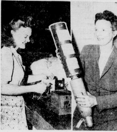
In addition to providing a descending medium for men and equipment, parachutes also carry bombs. They were used against the Japs in the South Pacific with deadly success. Left: An employee of a war plant in Stoughton, Mass., uses an X-ray machine to inspect bomb garachutes. Right: Another employee holds a 23-pound bomb attached to its parachute which is in the cylindrical container.
