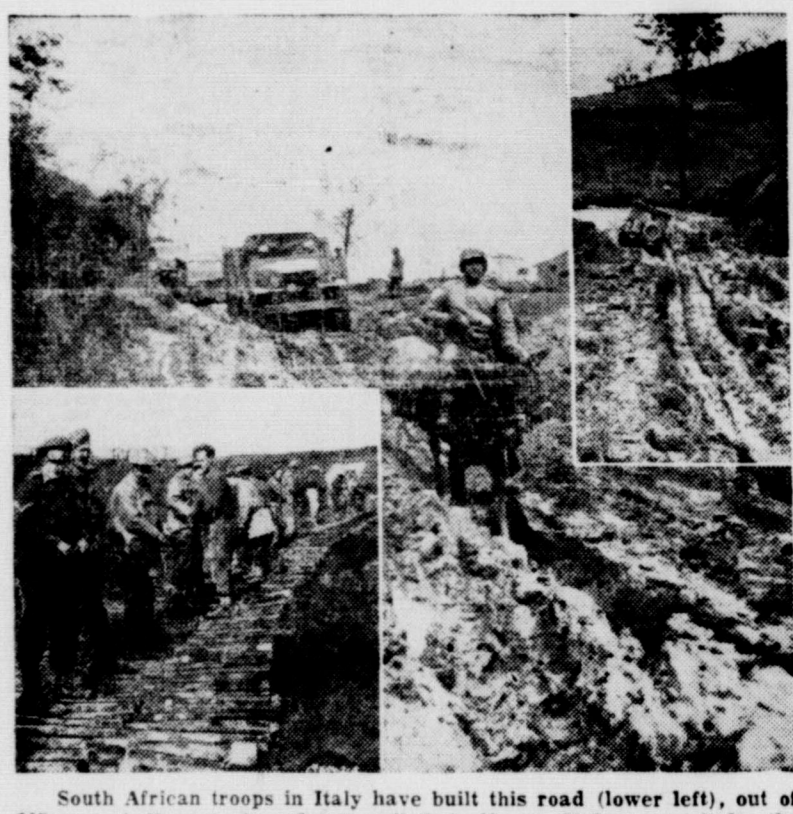
South African troops in Italy have built this road (lower left), out of 105-mm. shell cases, in order to pull their 40-mm. Bofors over it for the Fifth Army. Center—Mules are used to carry supplies south of Bologna when the mud gets knee-deep. Upper right—Hub-deep with mud, the Italian roads have slowed down supplies. In many sections it is necessary to fly in almost all material on account of impassable roads. Thousands of miles of roads are now being constructed by American engineers in France and Italy. While the construction takes time, many of the new roads are in operation.
