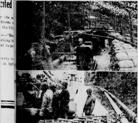
A pumping station, one of many set up along the pipeline carrying ital fuel oil in France. Upper photo shows station carefully camouflaged ainst air observation. Lower left, ship-to-shore line for unloading petrom from ships. Lower right, American engineers have laid this gasoline peline in France, five miles inland.
